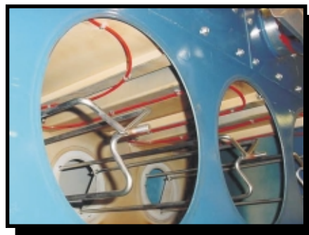
Image 4 - Firetrace Detection Tubing run above all of the filter cartridges
