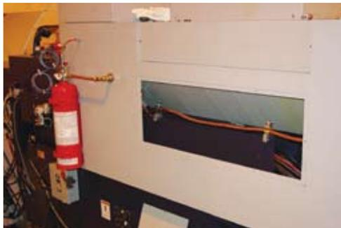
operate, so they can protect equipment that is powered down and left unattended. False discharges are unlikely because the tubing reacts only to heat and flame. The systems from Firetrace carry listings and approvals from UL, ULC, CE and other certifying agencies.
