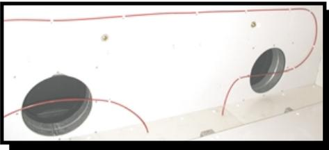
**Image 2** Firetrace tubing mounted across the exhaust vents.
