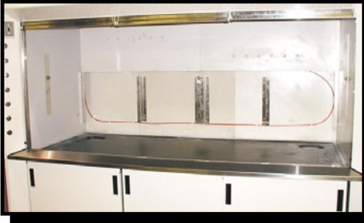
**Image 1** Firetrace tubing mounted in the baffles.
