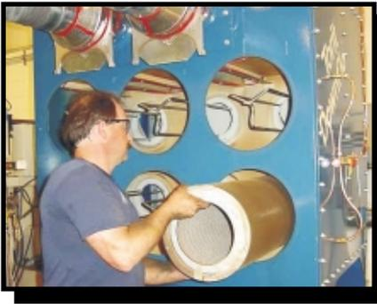
Image 2 - Filters installed on Dust Collector
