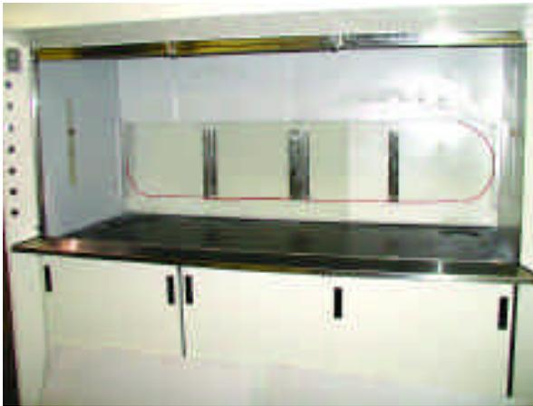
**Figure 2** Firetrace detection tubing mounted across the baffles of a fume cabinet.
